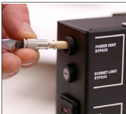
Installing Power Vent Bypass nonconducting slug. (Initially installed at the factory.)
