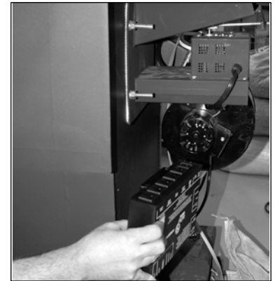
When mounting on rear wall, only mount on cool surface below 80 . If surface is too hot to touch, do not mount Power Module on it!
